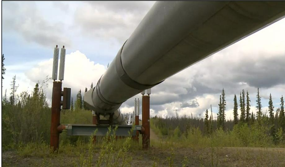
Abbildung 30: Alaska Pipeline mit Heatpipes (*As permafros thaws, protecting infrastructure becomes more important, 2021*)
