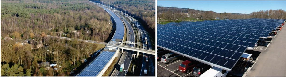
Abbildung 7: Links: Solarer Bahntunnel nahe Antwerpen/Belgien, 3,4 km, 50.000 m<sup>2</sup>, 3,3GWh/a. [newatlas.com/solar-rail-tunnel-completed/18881/](https://newatlas.com/solar-rail-tunnel-completed/18881/).
