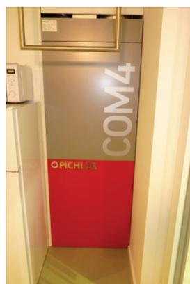
Abb. 103: PopUpDorms: Kombi-Wärmepumpe;
