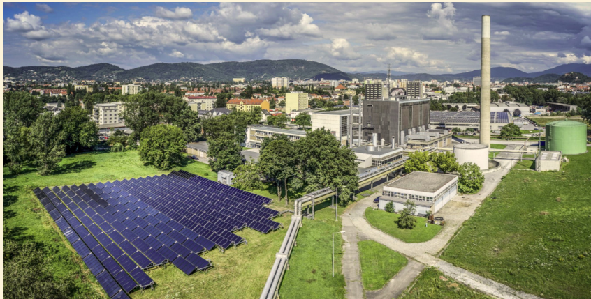
Collector field test at Fernheizwerk Graz, Austria:
