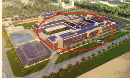
Solar COOLING and Hot Water by SOLID
