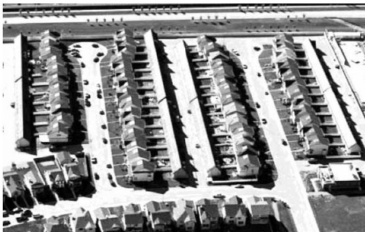
Figure 50: Okotoks complex (Canada)
