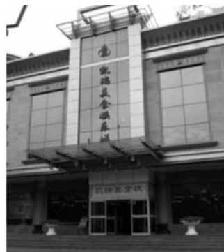
Shihezi Kai Rui Building
