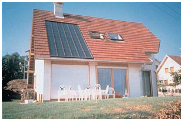
Figure 5: A French house with a direct solar floor system (Source: Clipsol, France). The daily storage for the space heating of the house is the concrete floor itself.
