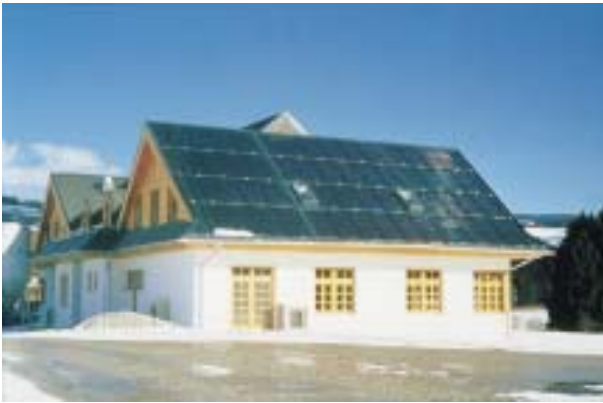
Figure 13: Roof-integrated collectors. The far left and far right section of the roof is a dummy. As they are the same colour it gives a uniform look to the roof as a whole. In this case two roof windows have also been integrated in the collector roof.
