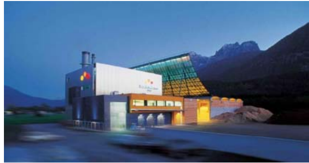
Figure 26: Solar assisted biomass district heating plant, Lienz, Austria
