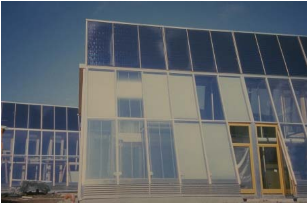
Figure 21: View of terraced houses
