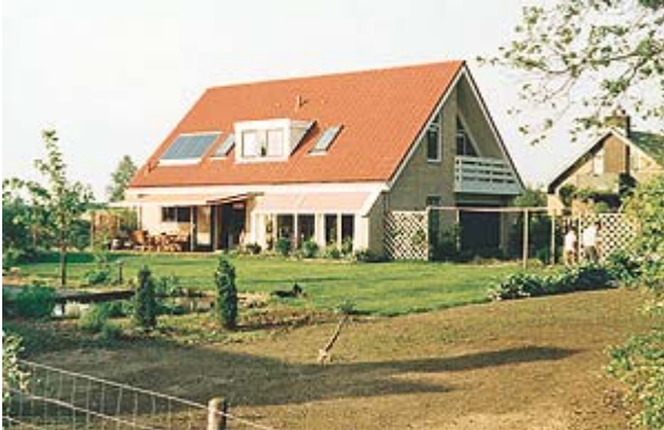
Figure 6: A Dutch house with a solar combisystem (Source: ATAG, The Netherlands)
