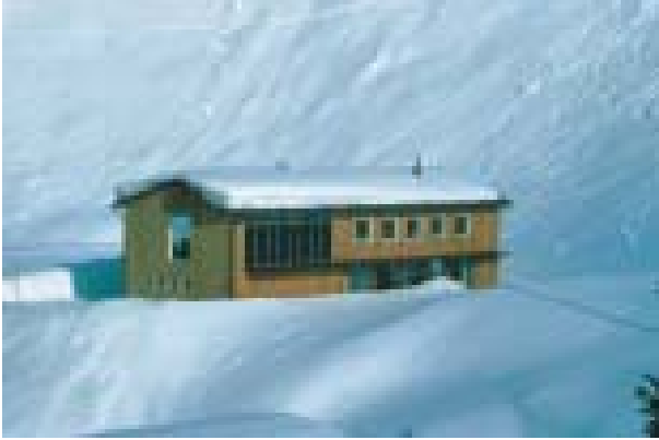
Figure 15: In regions with snow, facade-integrated collectors for solar combisystems have several advantages. No snow cover on the collectors and high irradiation on the façade due to the reflection of the snow (Source: AKS DOMA, Austria)
