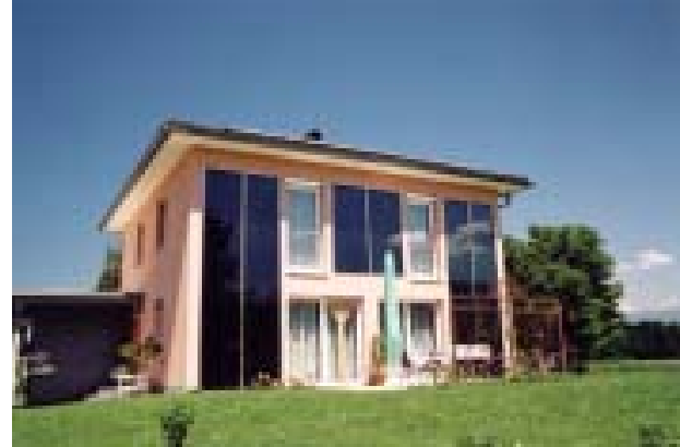
Figure 17: Solar heating system with 22.7-m 2 façade-integrated collector area for domestic hot water and space heating in a new single-family house.
