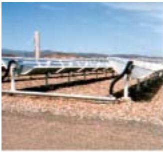
Fig. 18: Troughs can be connected in series and/or in parallel to form a larger collector array (picture source: AEE INTEC, Austria and CIEMAT, Spain)
