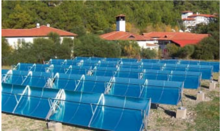
Fig. 16: 180 m 2 aperture area of parabolic trough collectors at a hotel in Turkey (picture source: SOLITEM, Germany)
