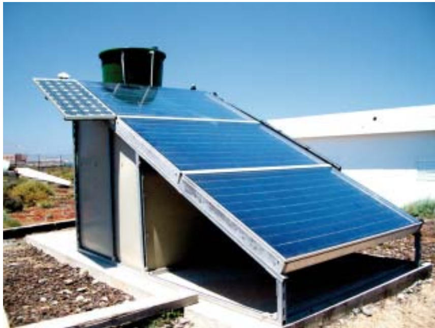
Double-glazed AR collector from ESE used in a solar driven desalination system installed December 2004 in Gran Canaria, Spain. The collectors and the desalination system are still in operation and have shown very good performance.
