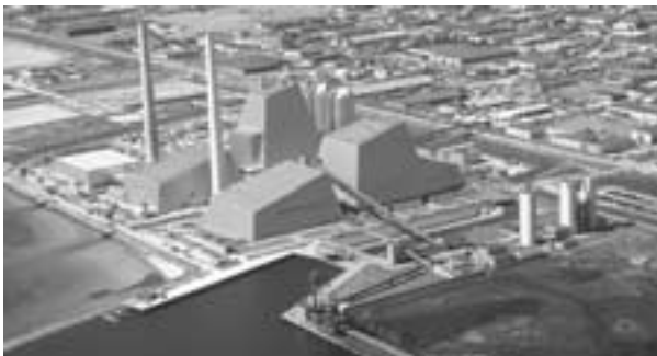
The Avedøre Power Station, south of Copenhagen, shows prize winning architecture. Avedøre 2 is the second unit. (Courtesy Thomas Scott Lund, Energi E2, Denmark)
