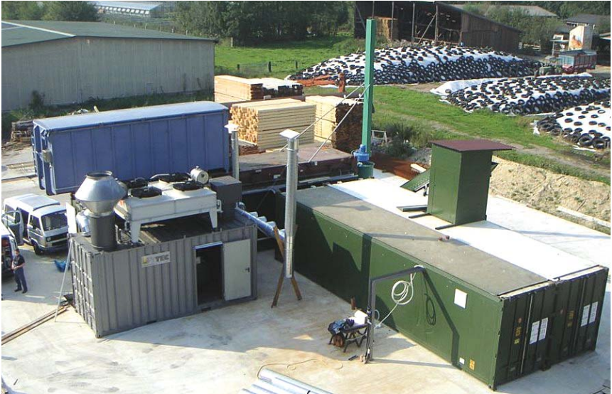
Figure 6: PyTec 50 t/d ablative pyrolysis demonstration plant
