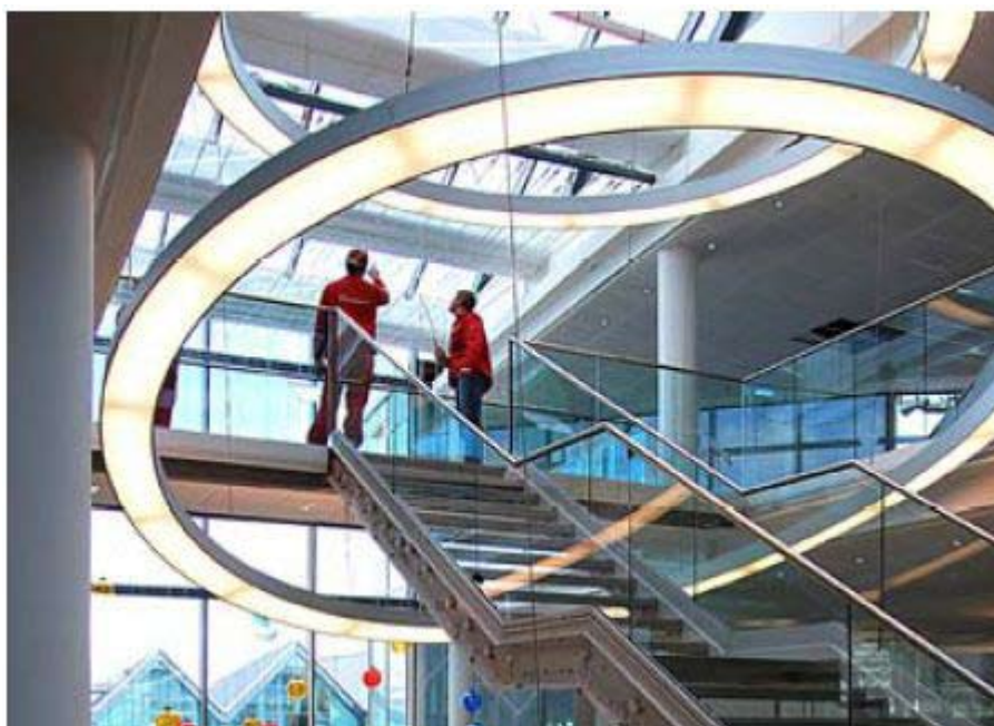
Optimised daylighting with LEDs for general lighting
