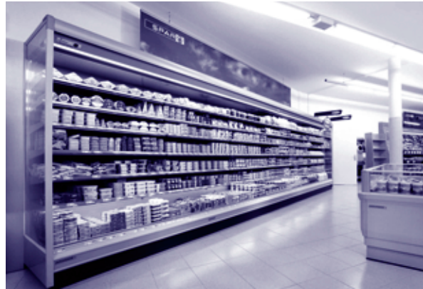
A supermarket refrigerator case uses heat pumps to minimise loss.
