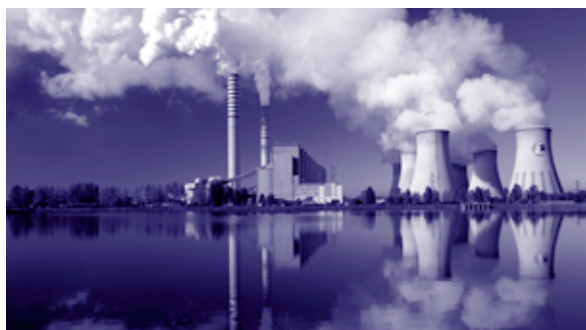
Poland's largest lignite-fired power plant, the 4320 MW Belchatow station, burns 35 Mt/year of lignite.
