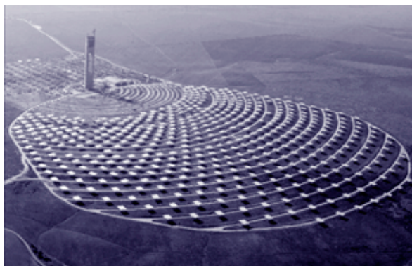
First commercial, 11 MW PS10 solar power tower plant (Seville, Spain).
