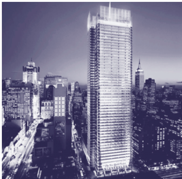
Ceramic tubes adjust daylighting in the New York Times building.
