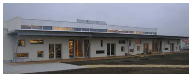
Figure 8 – Outside view of the Ziersdorf Kindergarten.
