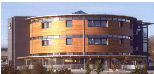
Figure 3 – Front view of the Christophorus Building
