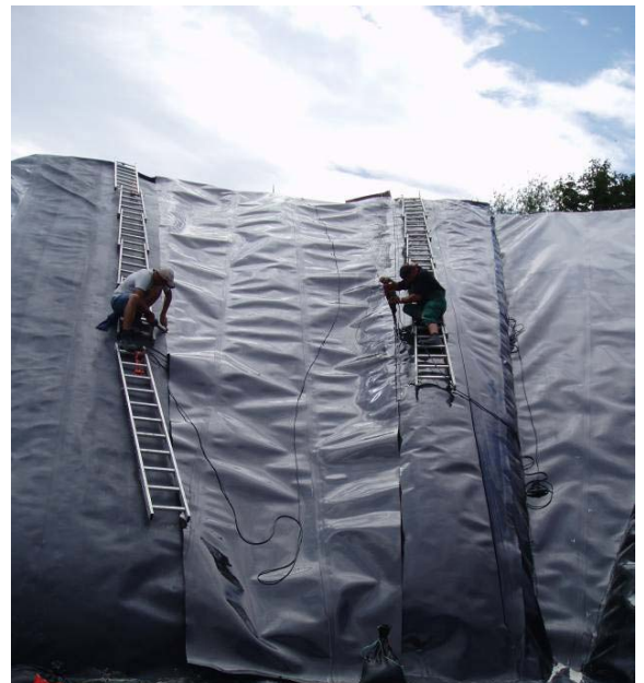
Polymeric liner installed in a seasonal thermal energy store (Eggenstein, Germany).
