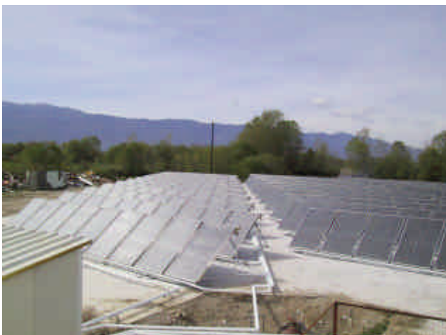
706 kW solar thermal plant for a dairy in Greece (sources: CRES – Centre for Renewable Energy Sources, Solenergy Hellas S.A.)
