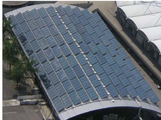
Fig. 3 Solar thermal plant, football stadium "UPC-Arena" in Graz, Austria (Source: SOLID, Austria)
