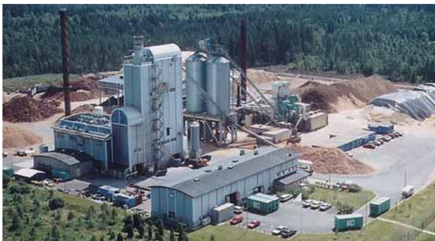
Biomass gasification plant with IGCC-Process at Vaernamo, Sweden.
