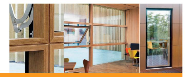
mental impacts. On account of the structural bonding of wood and glass, the windowpane also serves as reinforcing element. This facilitates the use of very slender wood frames and improves torsional stability.
