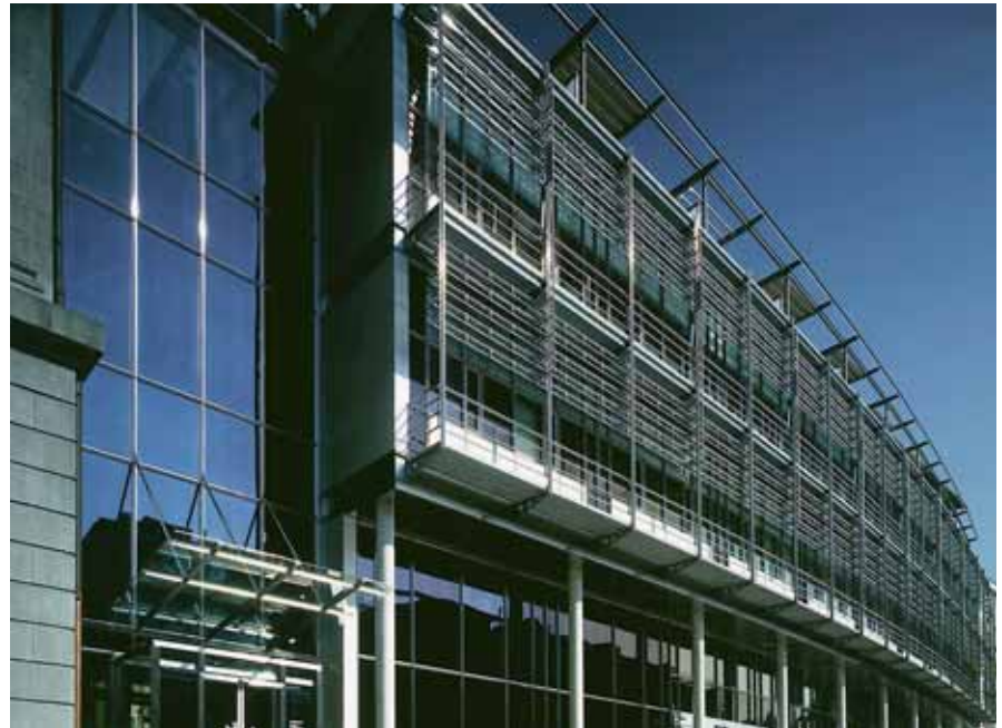
Schweizer Bankverein Biel: System using prismatic panels for light directing and sun shading.
