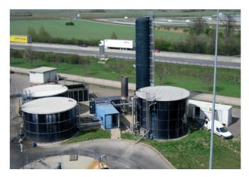
first time in Austria. Since 2007 a demonstration facility in Bruck an der Leitha has been purifying biogas to natural-gas standard at a rate of 180 m<sup>3</sup>/h and feeding up to 800,000 m<sup>3</sup> per year into the grid. The project reveals that purifying biogas to naturalgas standard is technically feasible, energy-efficient and economically profitable.
