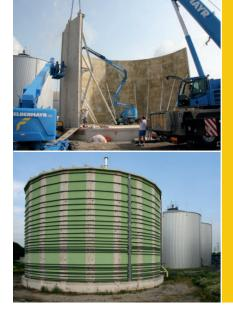
environmental advantages: 90 % less CO<sub>2</sub> is released during production. The resulting concrete is more resistant to acid and resists chemical attack much better than the material previously employed. It is no longer necessary to apply a coating to the inside of the digester; here again, material and expense are saved.
