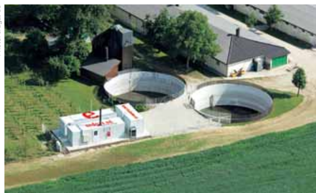
Photos: First grid-coupled biogas plant in Austria erdgas oö, Plant at Pucking operated by erdgas oö and OÖ Ferngas AG
