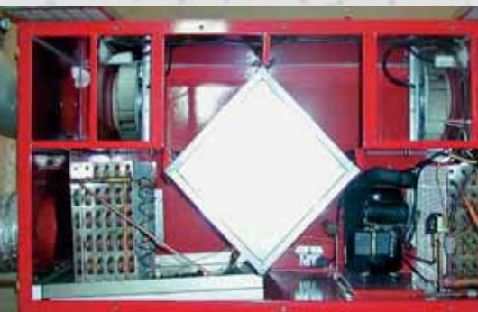
Ventilation unit with countercurrent heat exchanger and integrated heat pump.
