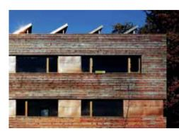
■ Passive use of solar energy South-facing passive houses are designed as solar houses. After the potentials of insulation and heat recovery have been exploited, the passive use of solar irradiation compensates about 40% of the remaining heat loss. To achieve this, windows are usually equipped with triple glazing and superinsulated frames. Thus, these windows let in more solar heat than is lost through them. An optimal solution should use south-facing glazing surfaces that are not shaded.
