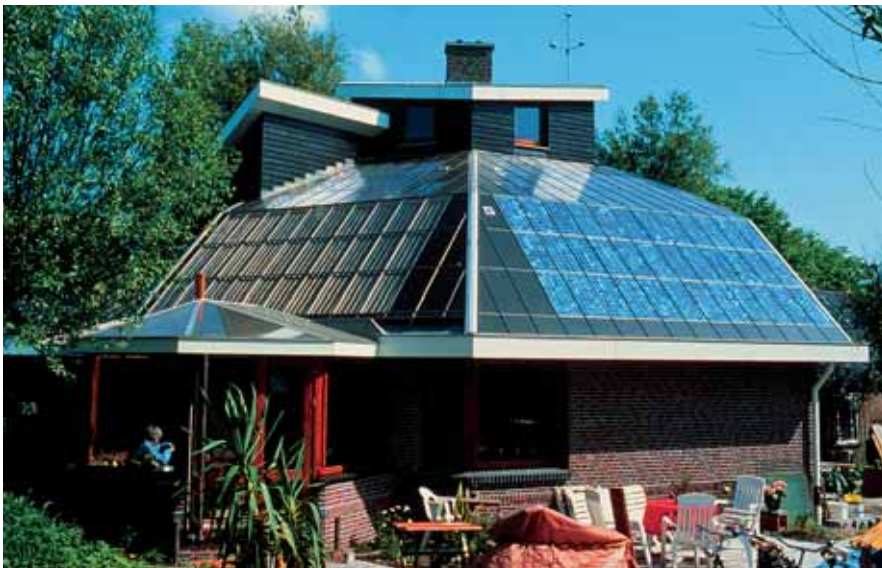
House with autonomous energy system in Woubrugge, Netherlands
