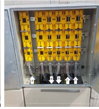
microgrid connection point
