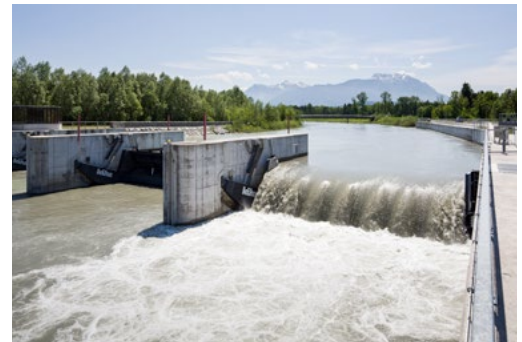
Stadtwerke Feldkirch, Illspitz power station; photo: Dietmar Walser
