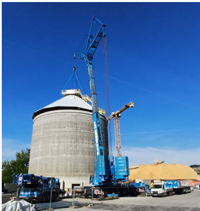
Biomass silo (exterior view), photo: Sappi Austria GmbH
