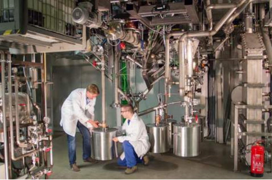
Lower part of the research plant without thermal insulation, photo: TU Wien
