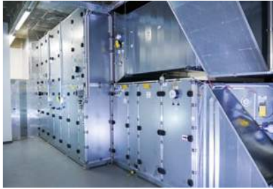
Ventilation system with heat and moisture recovery. Photos: Waldhör KG
