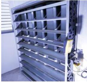
Ventilation system with heat and moisture recovery. Photos: Waldhör KG
