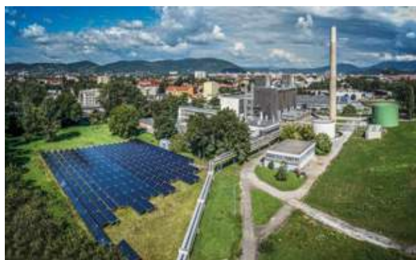
2014 installed field of solar collectors (2480 m 2 ) at the area of AEVG-Fernheizwerk Graz, Photo: S.O.L.I.D.
