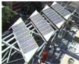
2. Inclined type module on roof
