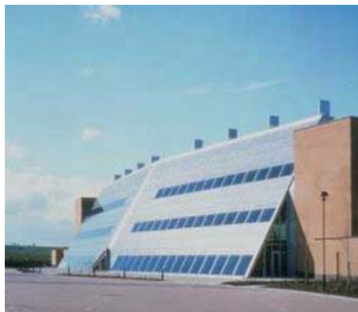
Abbildung 4.6: Well engineered Quelle: http://www.level1.nl/ECN
