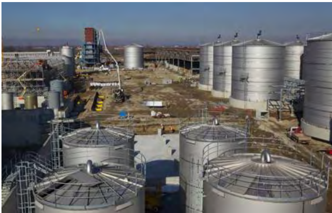
Figure The Mossi & Ghisolfi 40,000 t/y lignocellulosic EtOH plant under construction
