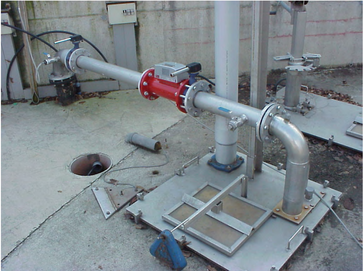
Photograph 6.8: Biogas flow meter of company ESTERS Elektronik, Type 005 GD 100 / with data processor GVPA-303-GDR, for measurements of the biogas flow from the storage to the other part (secondary digester) of the biogas plant.
