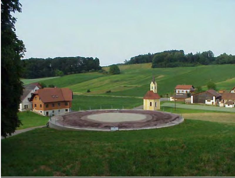
Photograph 6.7: Closed storage tank of digested material (concrete cover)
