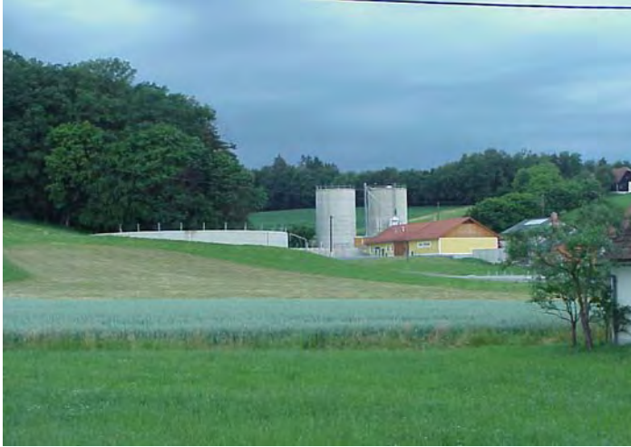
Photograph 6.1: Biogas Plant Paldau
