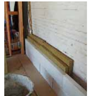
↑ Illustration 151 : Insulation by inside
