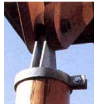
↑ Illustrations 390 and 391 : Wood frame - easy to disassembling
