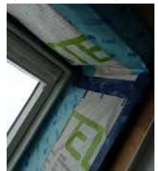
↓ Illustration 170: Air and water tightness of a frame
