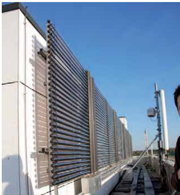
↓ Illustration 279 : Vacuum collectors.
