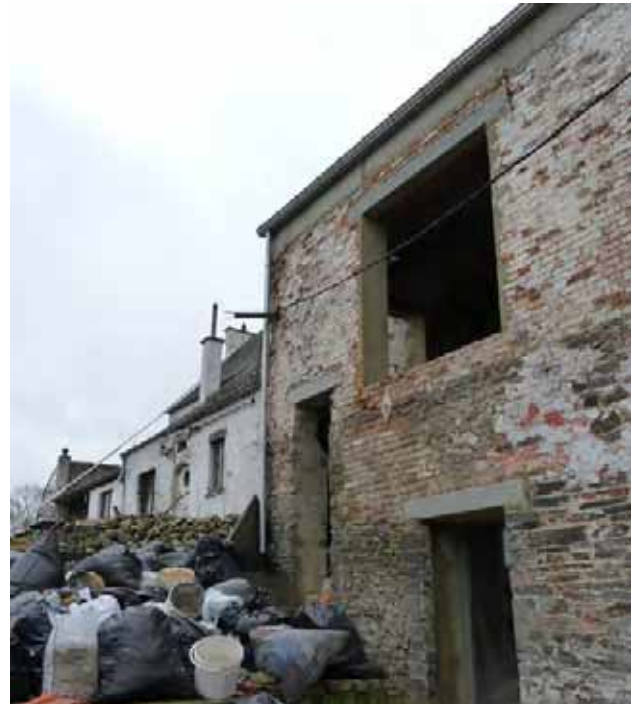
↑ Illustration 50 : Exemple of a large renovation
