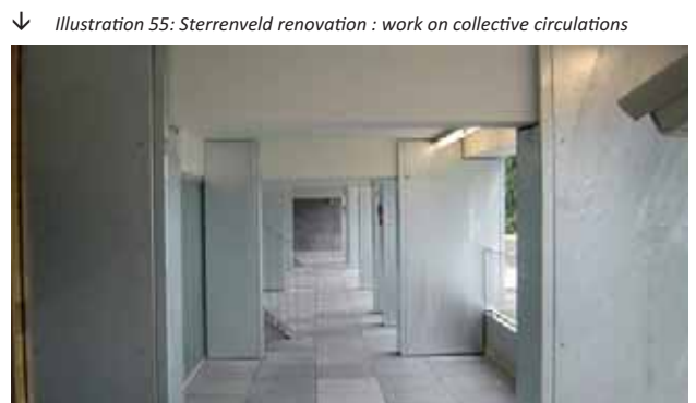
↓ Illustration 55: Sterrenveld renovation : work on collective circulations
