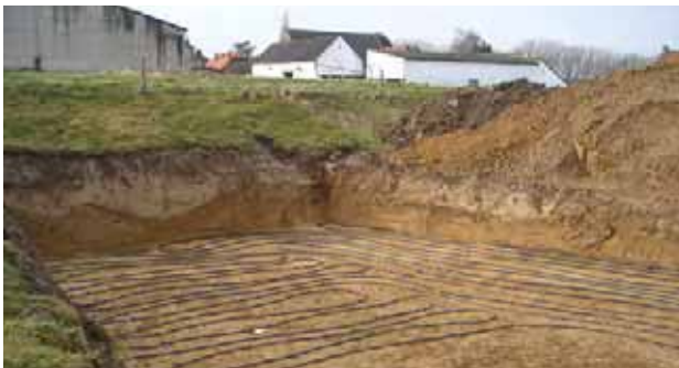
↑ Illustration 260 : Implementation of horizontal collectors.
