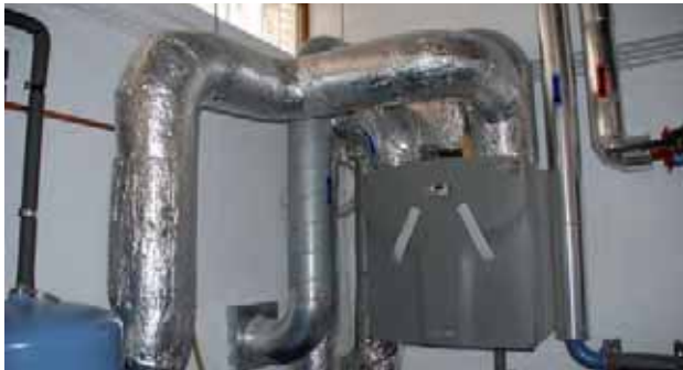
↑ Illustration 225 : Heat recovering - Balance ventilation system.
