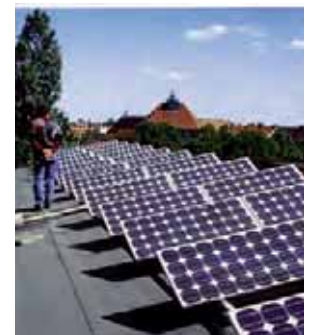
↑ Illustration 319: Installation on a flat roof
