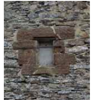
↑ Illustration 41: Vernacular massive wall
