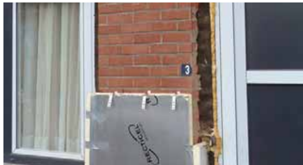
↓ Illustration 145: External insulation of an existing housing - Belgium
