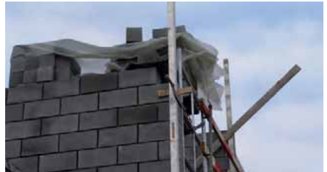
↑ Illustration 421 : Masonry work
