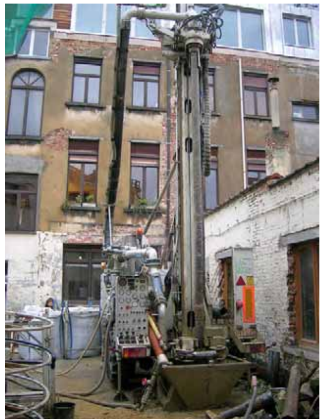
↑ Illustration 269 : Installation of heat pump - Provelo renovation - Brussel.
