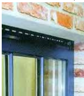
↑ Illustrations 92 and 93: Grilles for air intake in new frames
