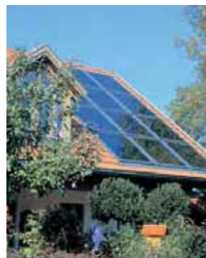
↑ Illustration 271 : Plane collectors.
