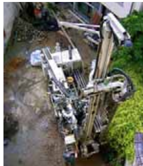
↑ Illustration 261 : Implementation of geothermic pump - vertical collectors.
