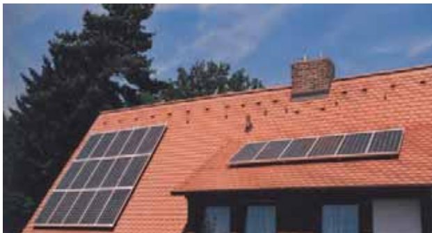
↑ Illustration 316 : The solar collectors, with different orientation, must be connected in parallel
