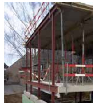
↑ Illustration 45: Steel frame work
