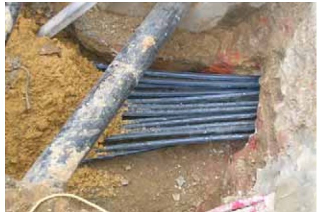
↑ Illustration 268 : Installation of heat pump - Provelo renovation - Brussel.
