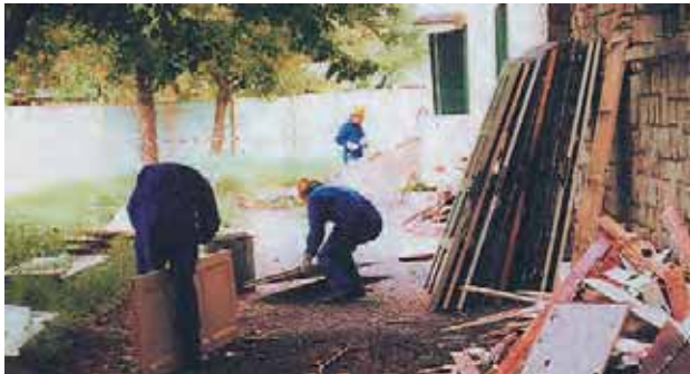
↑ Illustration 398 : Wood waste sorting on building site
