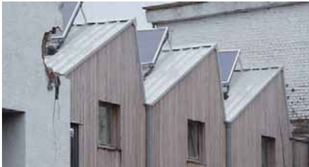
↑ Illustration 278 : Plane collectors in superposition of roof.
