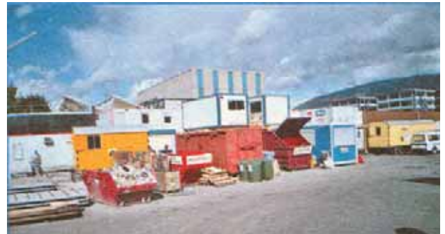
↑ Illustration 389 : Construction waste sorting on building site
