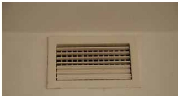
↑ Illustration 91: Installation of a ventilation system - grille
