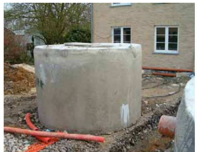
↑ Illustration 347 : Concrete water tank
