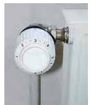
↑ Illustration 229 : Radiator valve.
