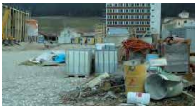
↑ Illustration 418: Production of waste on building site
