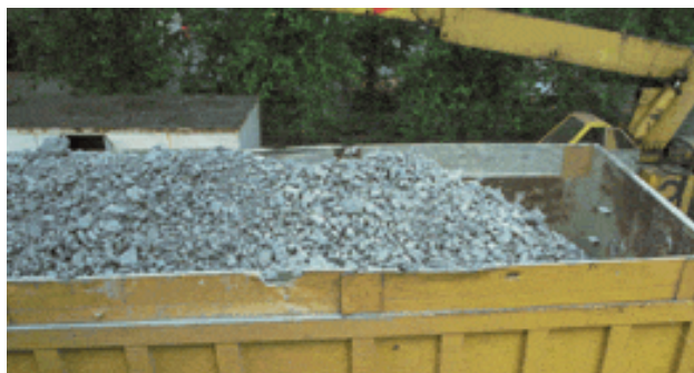
↑ Illustration 417: Production of waste on building site
