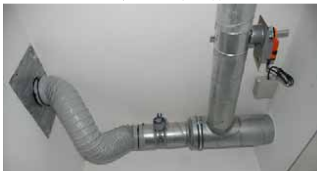
↑ Illustration 90: Installation of a ventilation system - pipes
