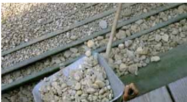
↑ Illustration 372 : Installation of gravel layer
