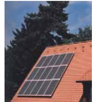
↑ Illustration 318: Installation on a roof
