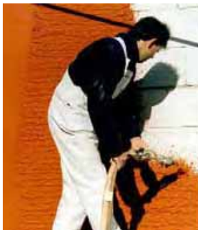
↑ Illustration 172: External coating on masonry
