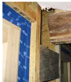
↓ Illustration 170: Air and water tightness of a frame
