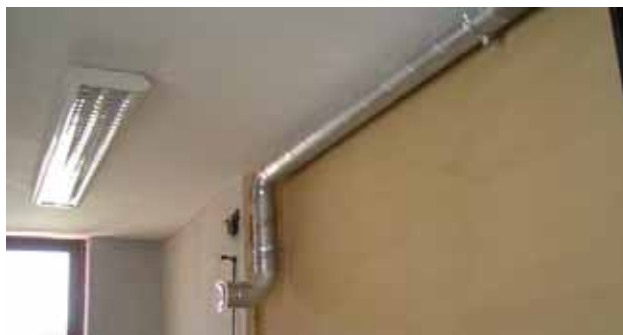
↑ Illustration 89: Installation of a ventilation system - pipes
