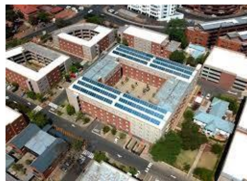
Wits Junction solar system is the largest solar thermal installation in Sub-Saharan Africa. It combines solar, co-generation and gas heating technologies, servicing 14 student residence buildings with one centralised hot water plant. Installation includes a 600m 2 heating plant with 10m 2 of collectors. (Source: Wits Junction/SOLTRAIN)
