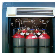
Example of an indoor fuel cell with indoor fuel storage (5 kW / 45 kWh solution).
