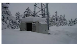
Example of an indoor fuel cell with outdoor attached fuel storage (1.7 kW / 120 kWh solution).
