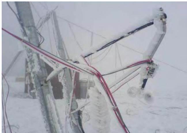
**Figure 4-1: A collapsed meteorological tower, likely due to heavy icing.**
