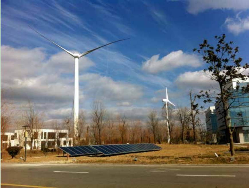
Figure 3. Wind-photovoltaics-storage intelligent micro-grid application project in Yancheng
