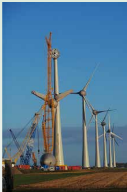
Figure 5. Enercon E-126 turbines being assembled along the dike at Noordoostpolder wind farm
