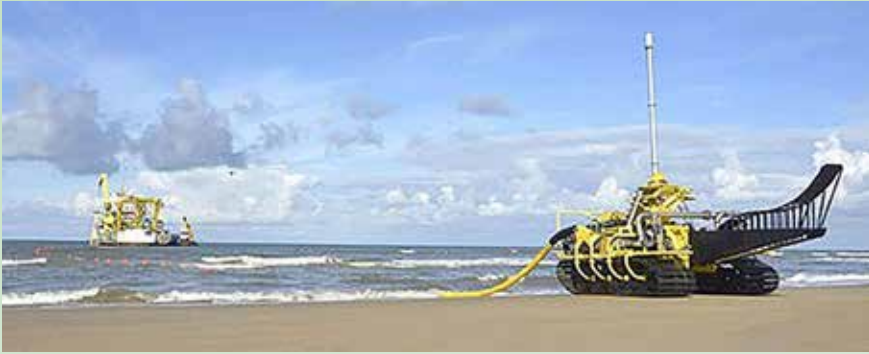
Figure 4. Arrival of the Luchterduinen cable at the beach near Noordwijk
