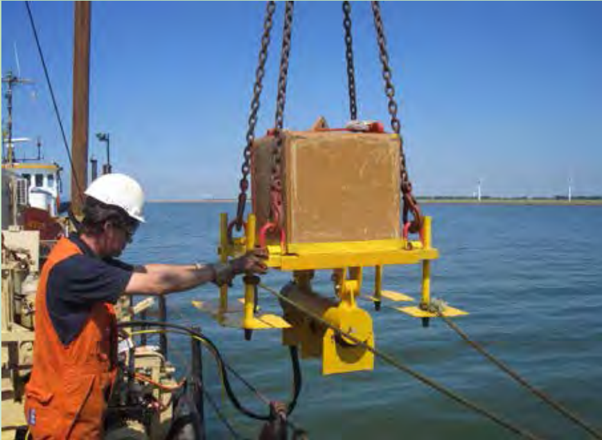
Figure 2. Equipment used for soil research to determine the interaction between soil and support structure and foundation
