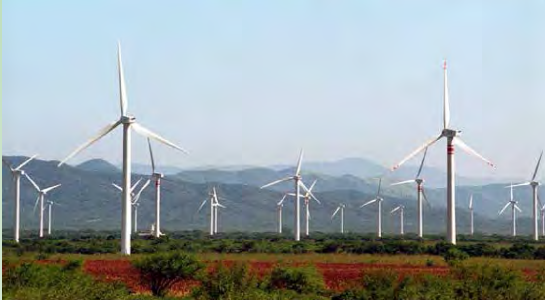
Figure 2. La Venta II 83.3-MW wind farm in the Isthmus of Tehuantepec, México
