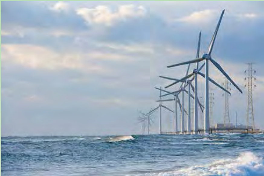
Figure 2. Wind Power Kamisu No. 2 offshore wind power plant in Ibaraki prefecture (Source: Komatsuzaki Urban Development Corporation)
