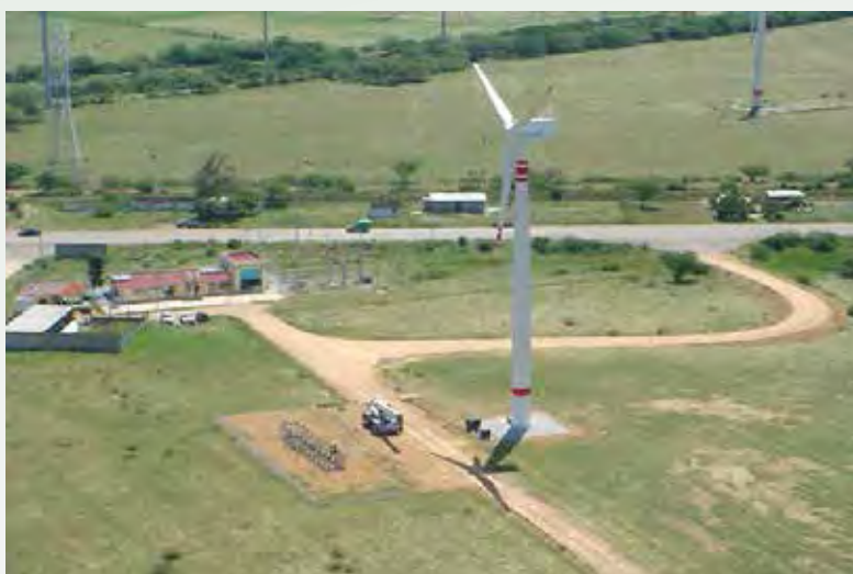
Figure 3. The Wind Turbine Test Center operated by the Instituto de Investigaciones Eléctricas
