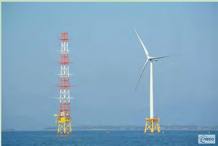
Figure 4. JSW 2-MW wind turbine and offshore measurement platform on the jacket and gravity hybrid foundation in Hibikinada offshore wind power demonstration project (Source: NEDO)
