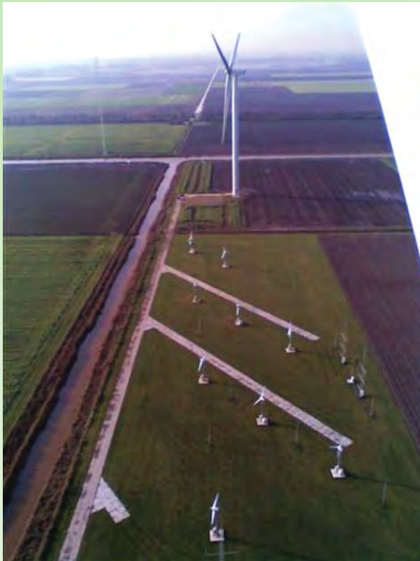
Figure 3. The nine small wind turbines at the ECN Wieringermeer test field are used to measure and model the wake in a wind farm (Photo: ECN)
