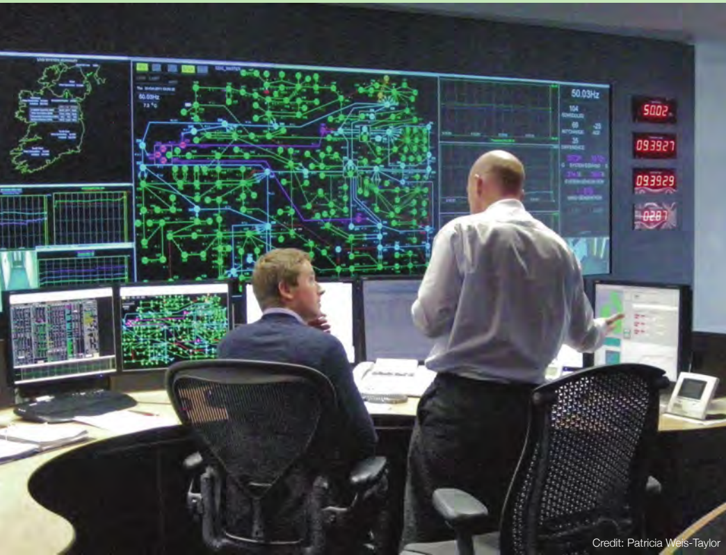
Wind energy production monitoring and control room, Dublin, Ireland
