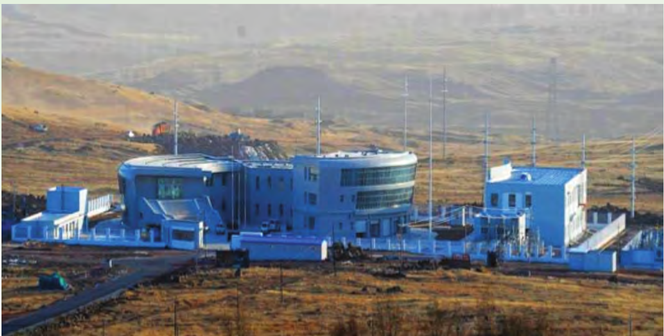
Figure 4. National Wind Power Integration Research and Test Center
