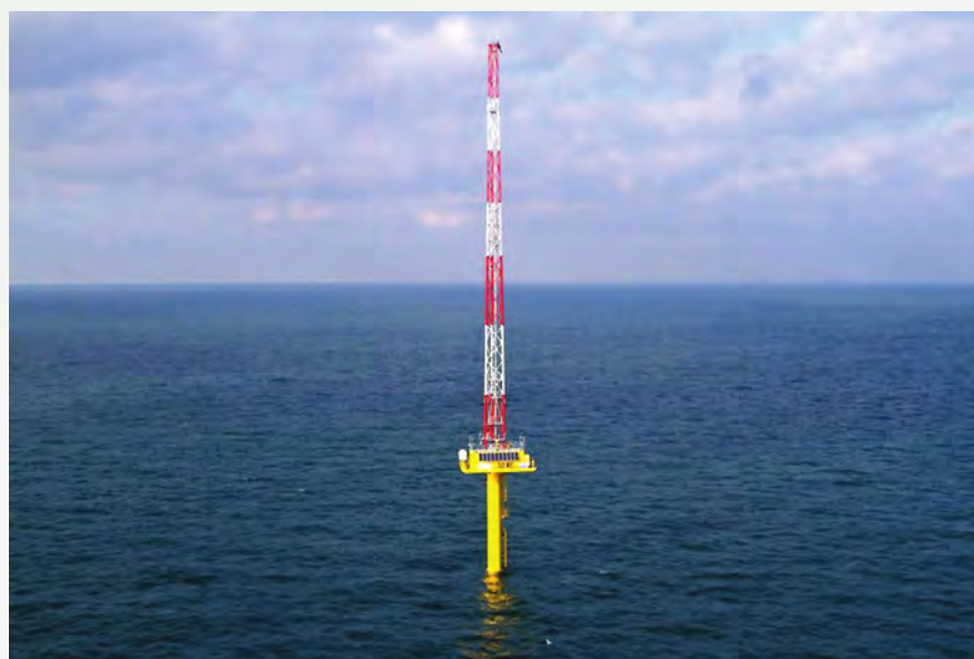
Figure 1. The RWE/Essent metmast, just after installation, without the booms
