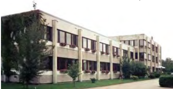
Before and after photos of a 1960s school in Schwanenstadt, Austria that was renovated to meet passive house standards.
