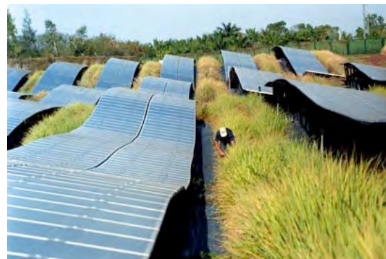
Solar field: Production of solar electricity (PV) and lemongrass essential oil in Reunion Island (Akuo Energy)
