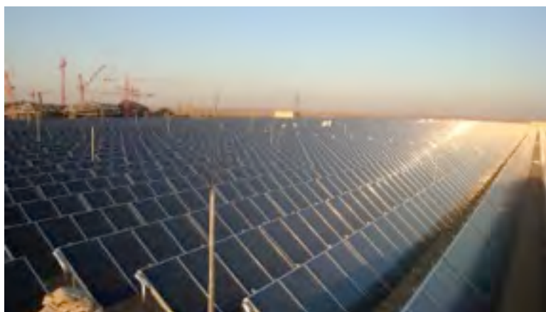
25 MW solar thermal plant at the Princess Noura bint Abdul Rahman University in Riyadh, Saudi Arabia
