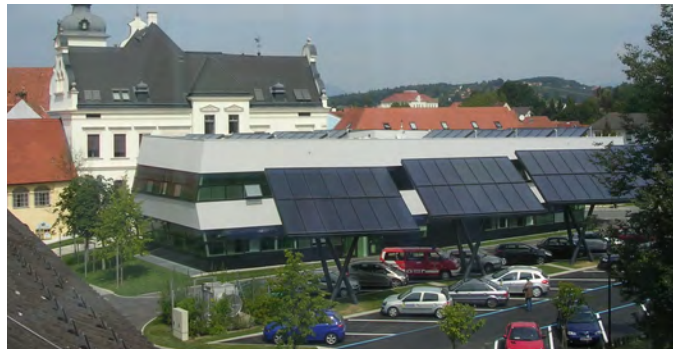
Figure 4. Solar heating and cooling installation at the Town Hall in Gleisdorf, Austria (304 m 2 flat plate collectors connected to 35 kW Yazaki chiller WFC 10 and a desiccant evaporative cooling system). (Source: AEE INTEC, Gleisdorf)
