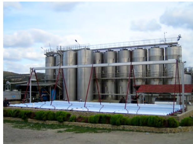
Figure 3. Solar cooling installation at the winery in Tunisia. In front: the Fresnel collector; the cooling of the wine storage tanks, shown in the background, is supported by the chiller, connected to the Fresnel collector.
