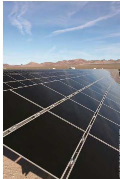
CdTe Thin Film Utility-scale PV, 58MW, Copper Mountain ; Nevada, USA, Sempra Energy
