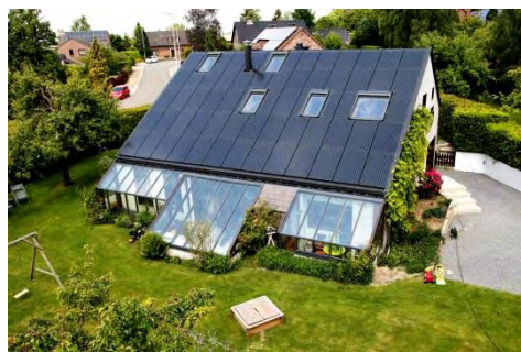
Tailor-made BIPV modules, ISSOL, Belgium
