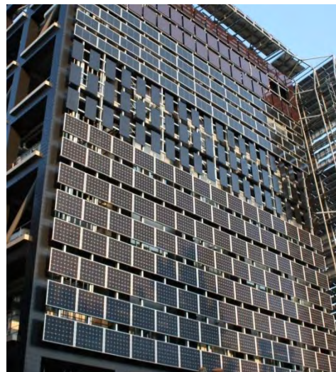
BIPV System in Japan, Courtesy of RTS Corporation
