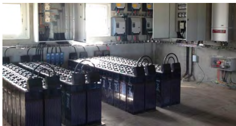
AC coupled PV/Diesel/Batteries Hybrid system implemented at Isona (Lerida), Spain by Granjes Pereto
