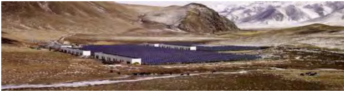
Figure 4.2.3-2 : Photo of 2 MW PV station with battery in Yushu County
