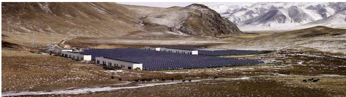
China, Yushu Valley, 2 MW PV Plant – Courtesy of Lu Fang.
