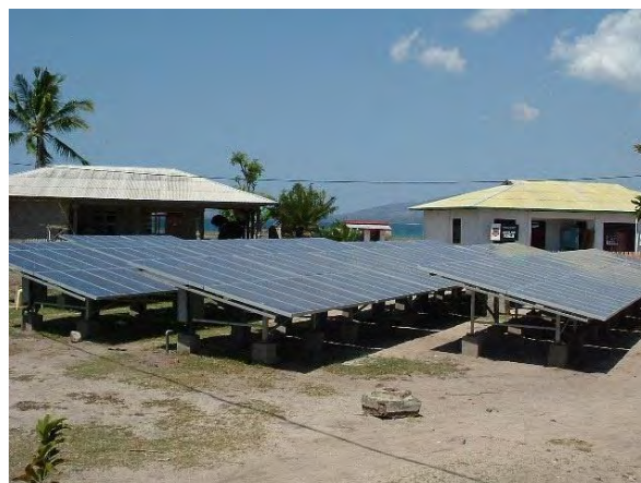
Figure 1: Pomelo, Indonesia, 24kWp, 20-kWh battery, 125-kVA genset (photo: TRANSENERGIE)
