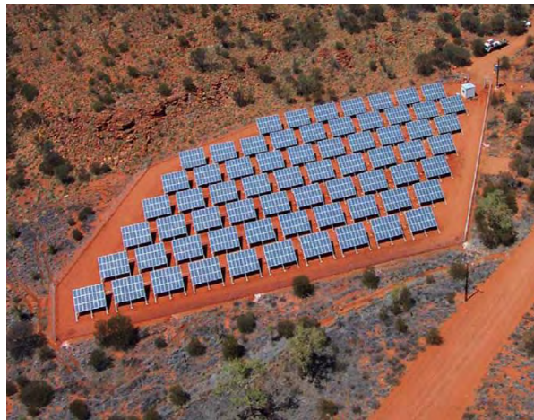
Figure 2: King's Canyon, Australia, 225kWp, three gensets operating continuously, Utility-operated 11-kV distribution network (photo: NOVOLTA Pty)
