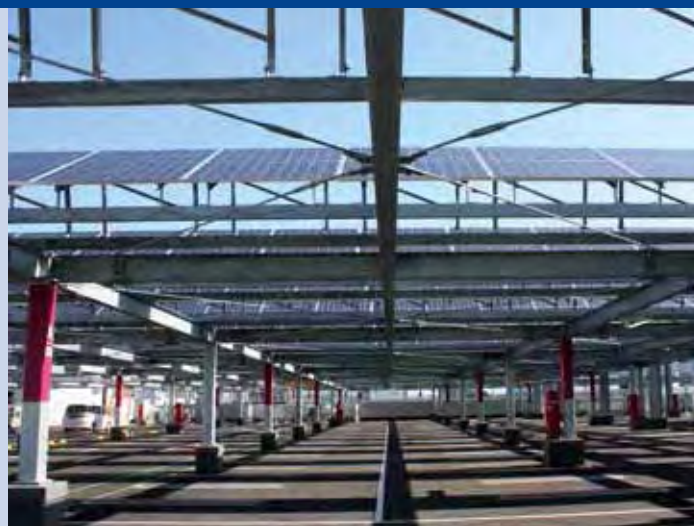
Fig. 2 - AEON Mall Makuhari New City (Mihama Ward, Chiba City, Chiba Prefecture). 242-W multicrystalline silicon PV module (Kyocera). Total: 1,75 MW, of which, parking area: 1 MW.
