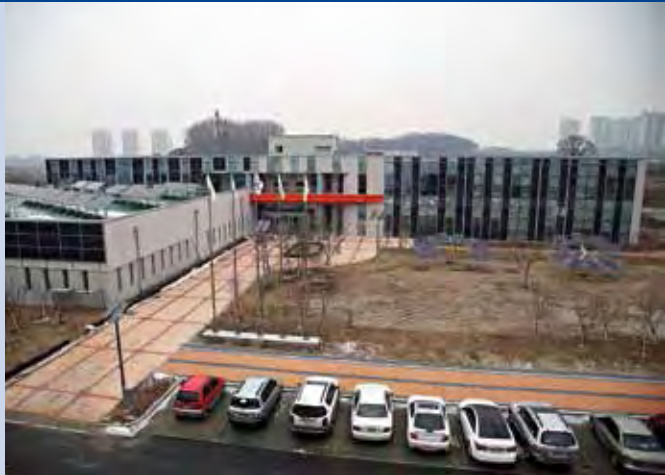
Fig. 1 - PV test-bed (Chungcheong region), Jincheon-gun, Chungcheongbuk-do, Korea.
