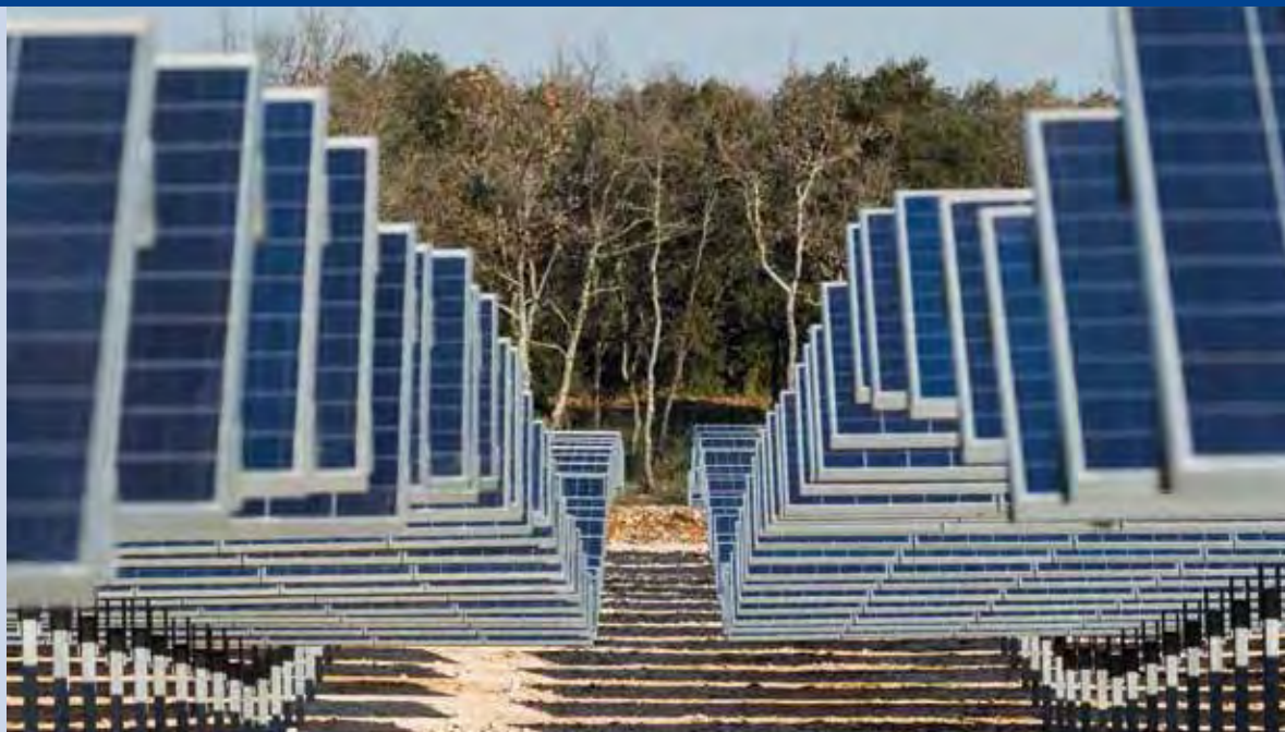
Fig. 2 – Photovoltaic power plant with horizontal single-axis tracker, 4,7 MW, Vallérgues (Gard Dpt), Urbasolar/Exosun (Photo: Christophe Ruiz).
