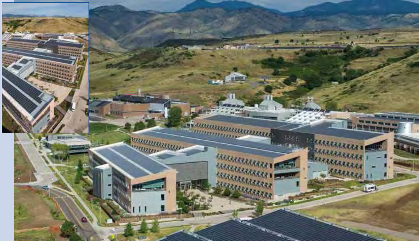
Fig. 3 - 2014 NREL South Table Mesa Campus. Aerial view of the RSF, S&TF, and ESIF, at the National Renewable Energy Laboratory (NREL), South Table Mesa campus (STM) Aerial view of the National Renewable Energy Laboratory (NREL), South Table Mesa campus (STM). (Photo: Dennis Schroeder / NREL).
