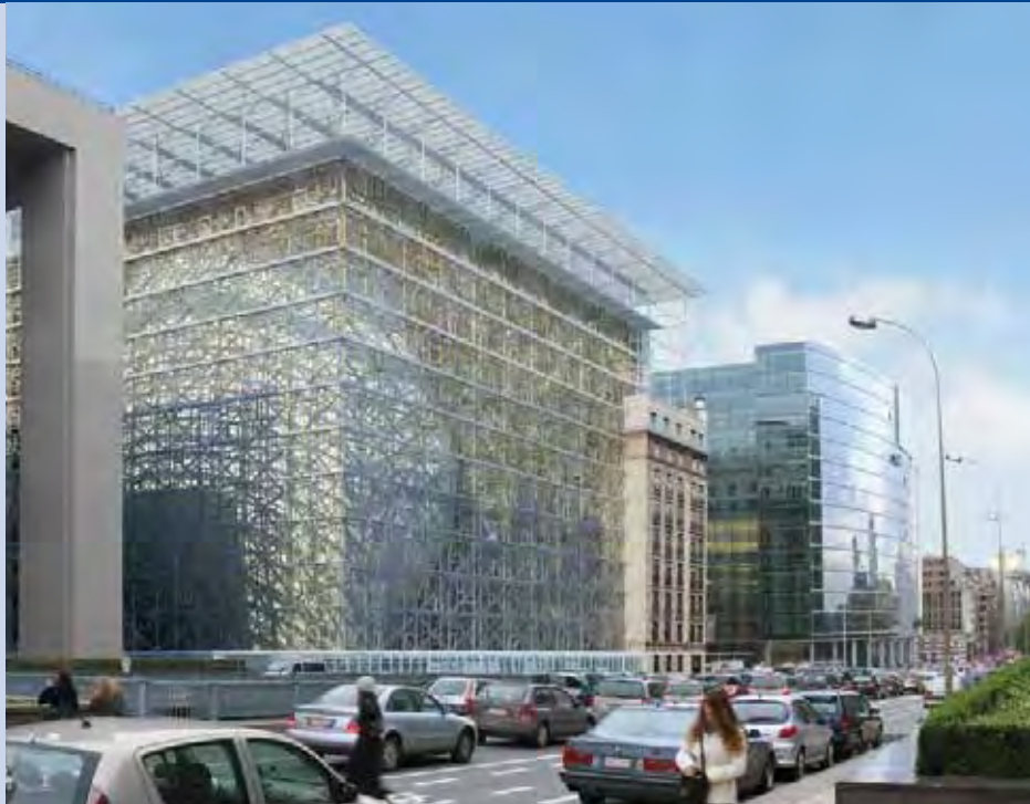
Fig. 1 - The new European Union council headquarters in Brussels. An umbrella of photovoltaic panels for the electricity production covers both the modern and the historical parts; symbolizing the link with the present, the past and the future.
