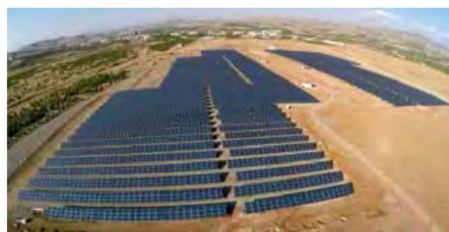
Fig. 1 - The largest PV system in Turkey with the installed capacity of 5,3 MW in Malatya.
