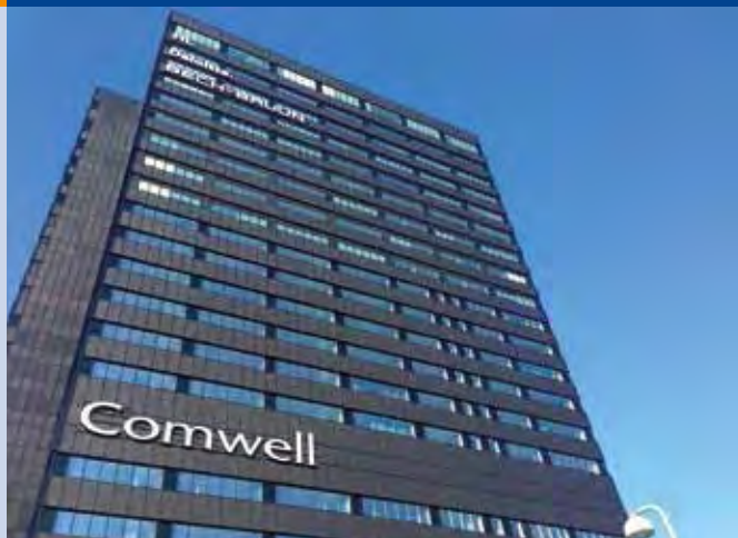
Fig. 2 - Aarhus City Tower. The system is produced by the Danish company, Racell SAPHIRE, and integrated as a 1 800 m 2 BIPV with a maximum power of 250 kWp. The building is fulfilling the energy performance building directive 2015. In the design phase, the focus was on architectural design, façade integration and energy production.
