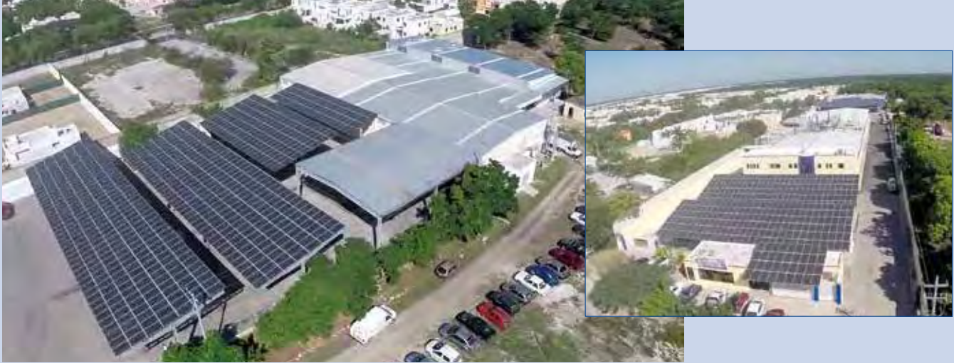
Fig. 1 - 324 kWp PV system installed in the parking lot of a snack factory in Merida Yucatan (Photo: CONERMEX).
