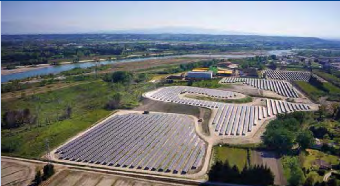
Fig. 3 – Photovoltaic power plant built on brownfields, 7 MW, Chateaurenard (Bouche-du-Rhône Dpt), La Compagnie du Vent/ Mydrone.fr (Photo: Lionel Barbe).
