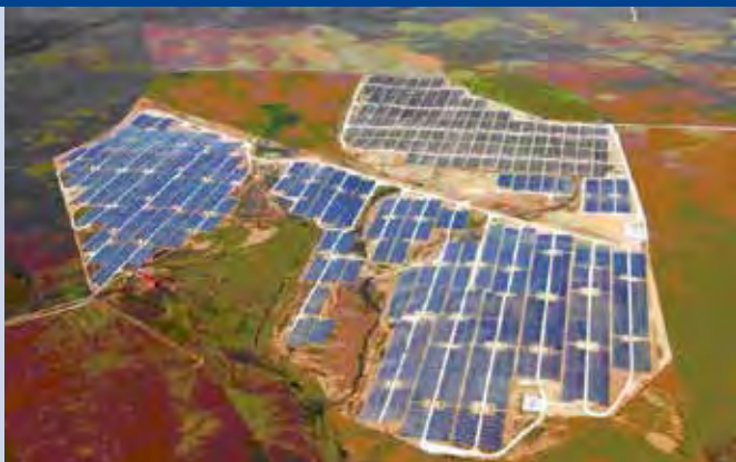
Fig. 1 - PV plant from ATERSA, 30MW, one axis horizontal, c-Si technology in Cáceres, Spain.
