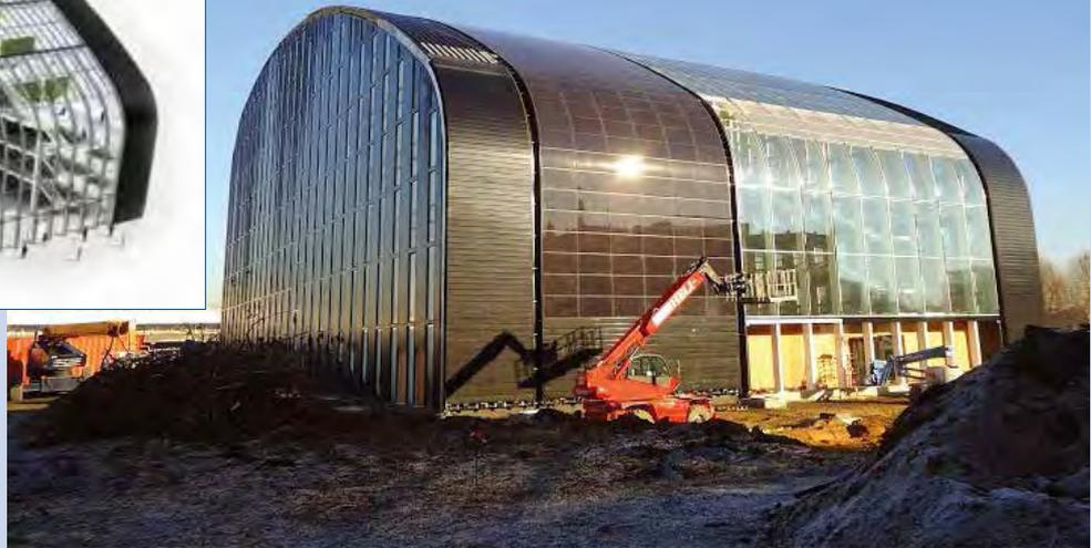
Fig. 1a & Fig. 1b - Bruxelles Environnement. The new Brussels Environment and Energy Administration Headquarters will be the largest passive office building in Europe and will include 700 m<sup>2</sup> of BIPV ISSOL modules (Photos: Copyright CEPEZED, ISSOL for Fig. 1a and ISSOL for Fig. 1b).
