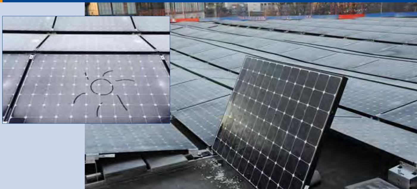
Fig. 4 - PV installation at Powerhouse Kjørbo, delivered by Direct Energy. The system has a capacity of 310 kWp (See also [www.powerhouse.no](http://www.powerhouse.no)).
