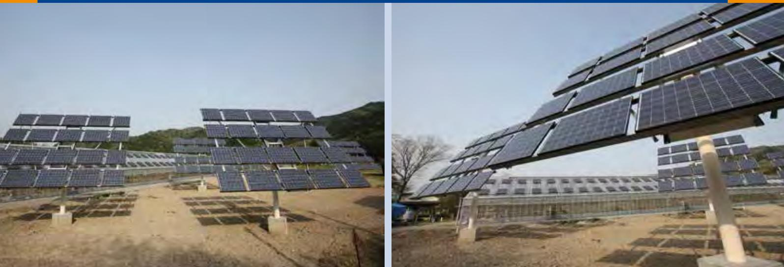
Fig. 3 - Fujipream's Experiment Farmland (Himeji City, Hyogo Prefecture) Tracking PV Systems: 30 kW, Greenhouse: 20 kW Fujipream (mc-Si).
