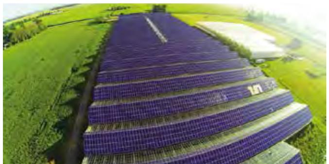
*Fig. 1 - At Vine Fresh Produce Project is the largest rooftop installation in Ontario under the FIT program (2,3 MWp). This project is currently the largest system in the world with an Enphase micro-inverter.*
