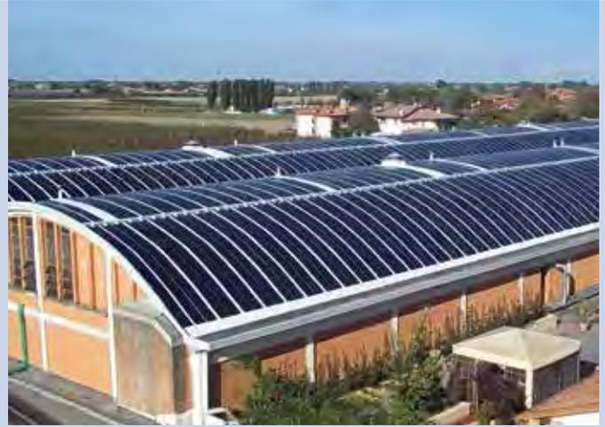
Fig. 2 - 123 kWp PV plant at Argenta (FE), using DERBISOLAR flexible modules (thin film on flexible support) (Photo: GSE, Gestore del Sistema Elettrico).
