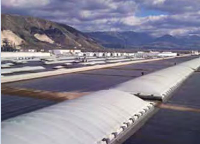
Fig. 1 - 1 544 kWp PV plant at Nola (NA), using General Solar Flexible Modules (thin film on flexible support) (Photo: GSE, Gestore del Sistema Elettrico).
