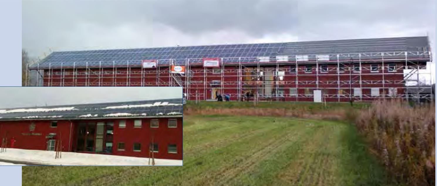
Fig. 1 and 2 - PV installation at Høgskolen i Hedmark, Avdeling Evenstad. 70 kWp system supplied by FusEn AS.
