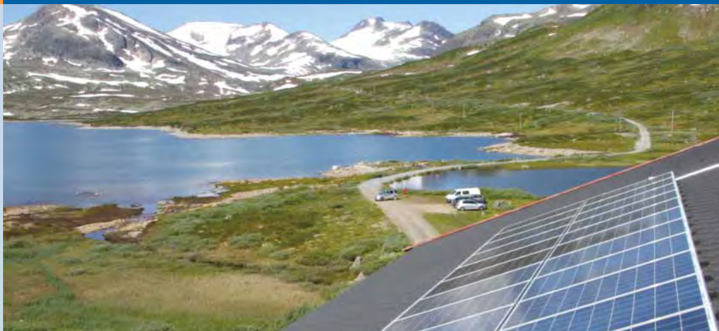
Fig. 2 - PV installation at Tyinholmen lodge in the Norwegian mountains. With 22 panels, approx 6 kW, supplied by REC.
