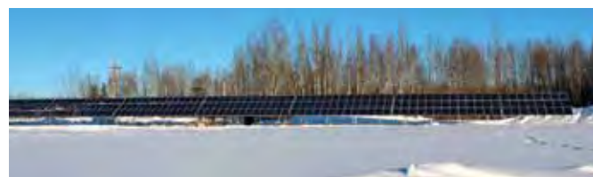
Fig. 2 - Fort Simpson is Northwest Territories Power Corporation largest diesel-powered community. This 61 kilowatt system (the largest North of 60 degrees in Canada) will help displace 15 000 litres of fuel annually and provide up to 8,5 % of the village's minimum power requirements during the summer (Photo: Skyfire Energy).
