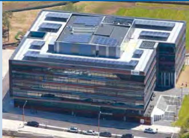
Fig. 3 - 5 Murray Rose Avenue, Olympic Park, Sydney. The 130,5 kWp commercial office rooftop PV system was used to achieve Peak Demand Reduction and Emissions Reduction credits towards a 6 Star Green Star certified office rating. The PV system is also a significant part of the 5 Star NABERS Energy target for building operation (Photo: The GPT Group).
