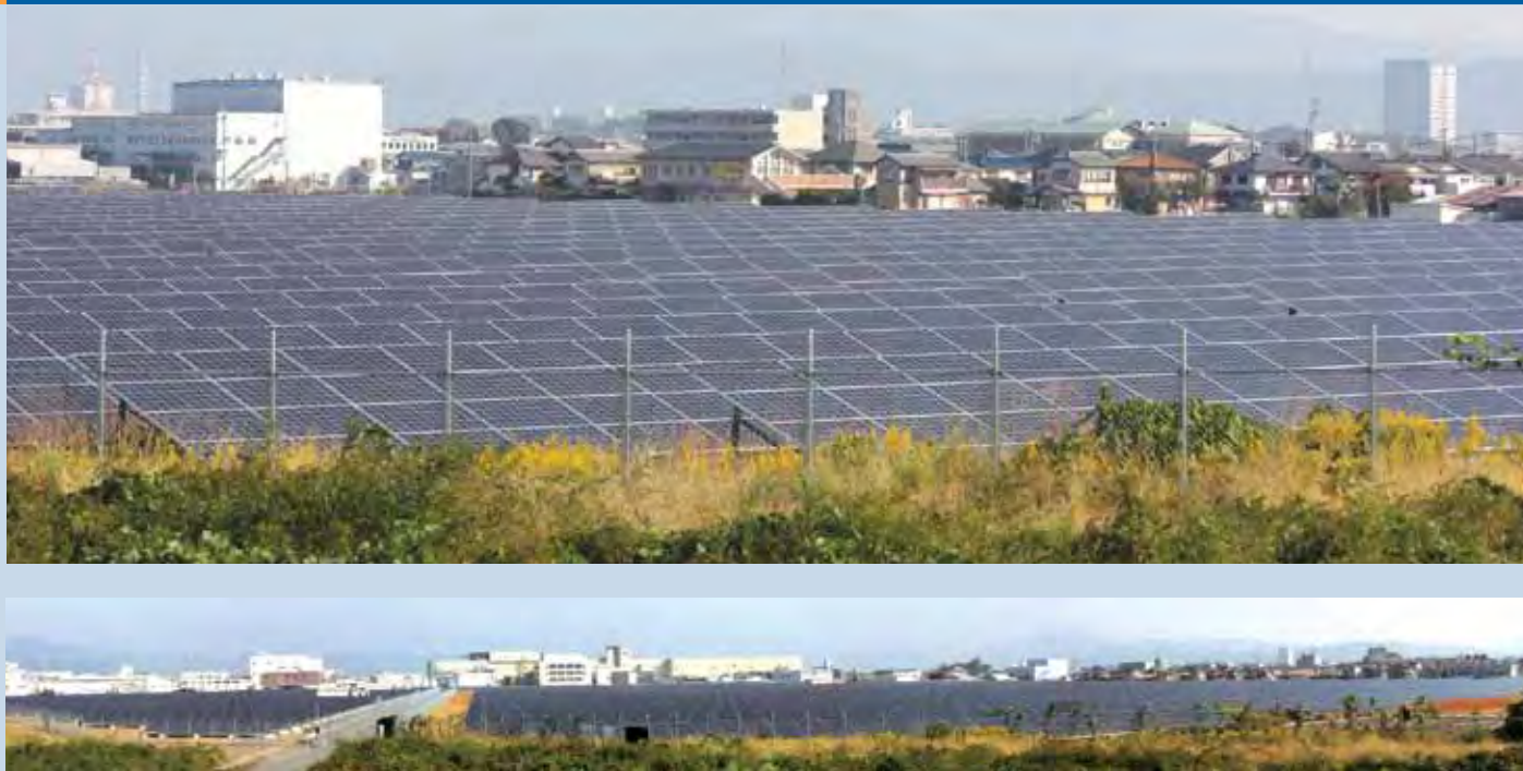
Fig. 2 – SoftBank Kyoto Solar Park (Fushimi-ku, Kyoto City, Kyoto Prefecture), 4,2 MW, Multicrystalline Silicon PV module by Kyocera.
