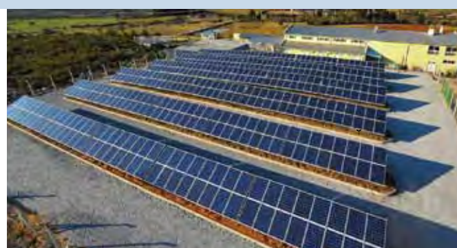
Fig. 4 - 105 kW grid-connected PV system in Muğla, Turkey.
