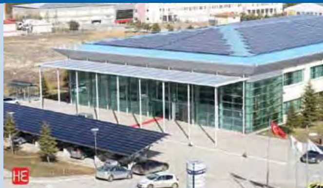
Fig. 2 - 420 kW grid-connected PV system in Ankara, Turkey.
