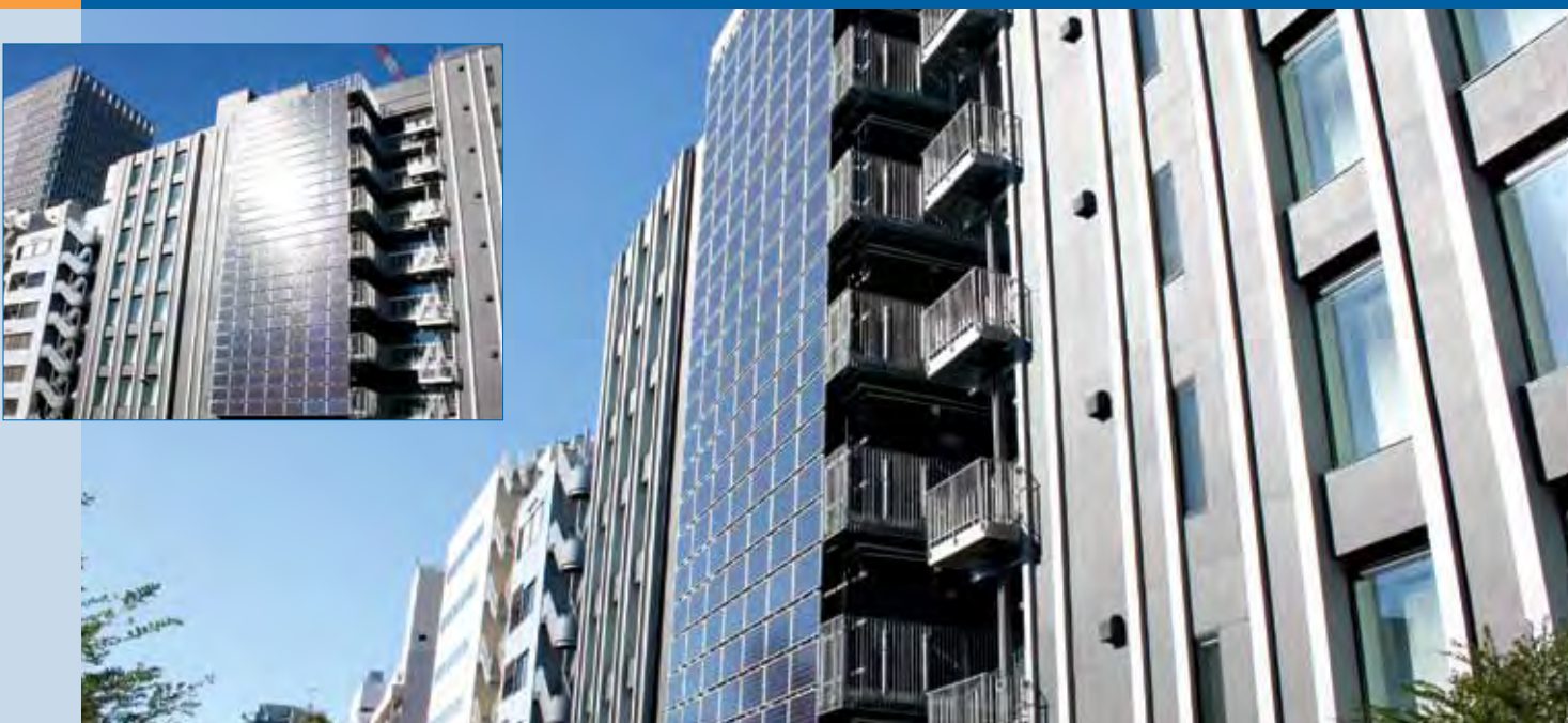
Fig. 3 - Kyobashi OM Building (Chuo-ku, Tokyo), 42 kW, Multicrystalline Silicon PV module.
