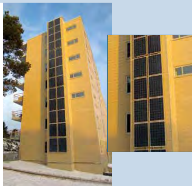
Fig. 3 - Façade mounted PV in the city of Göteborg (Photo: Energibanken).
