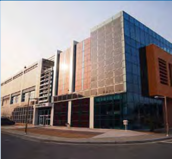
Fig. 1 – 111,2 kW BIPV system located at the Climate Change Research Building of the National Institute of Environmental Research, Incheon, Korea.
