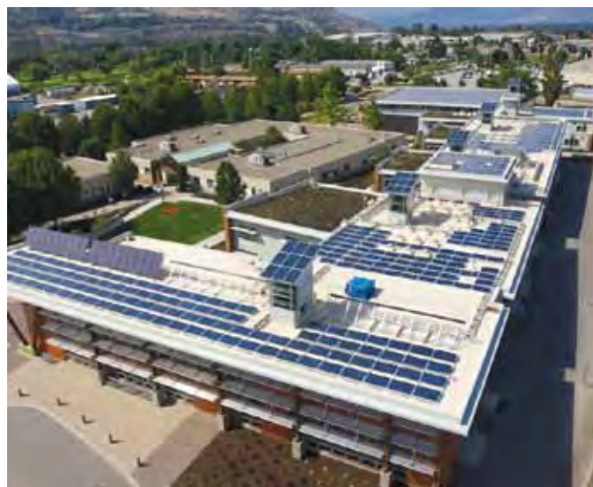
Fig. 1 - A 260 kilowatt solar PV rooftop system installed at the Okanagan College in British Columbia to meet the ambitious target for the living challenge and help train students in green construction practices (Photo: Skyfire Energy).
