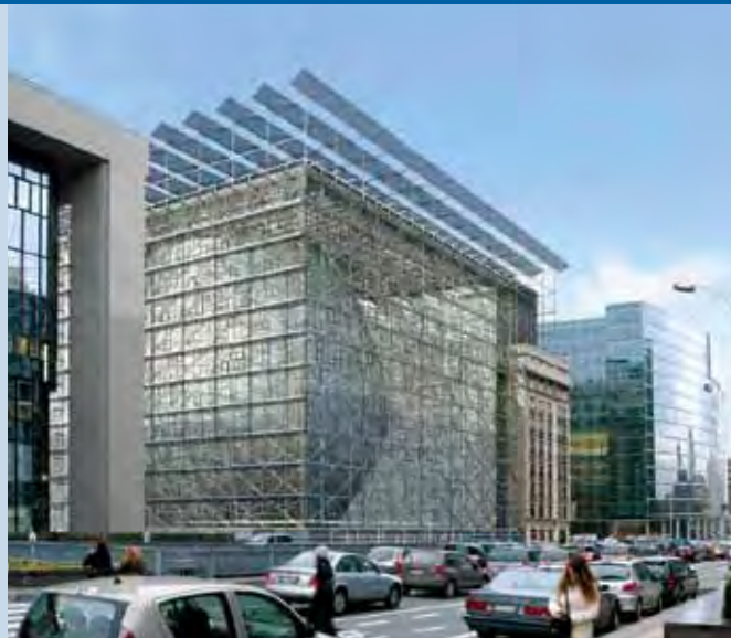
Fig. 4 – European Headquarters: Both the modern and the historical parts of the European Commission's new building, currently in construction, will be covered by an umbrella of photovoltaic panels.
